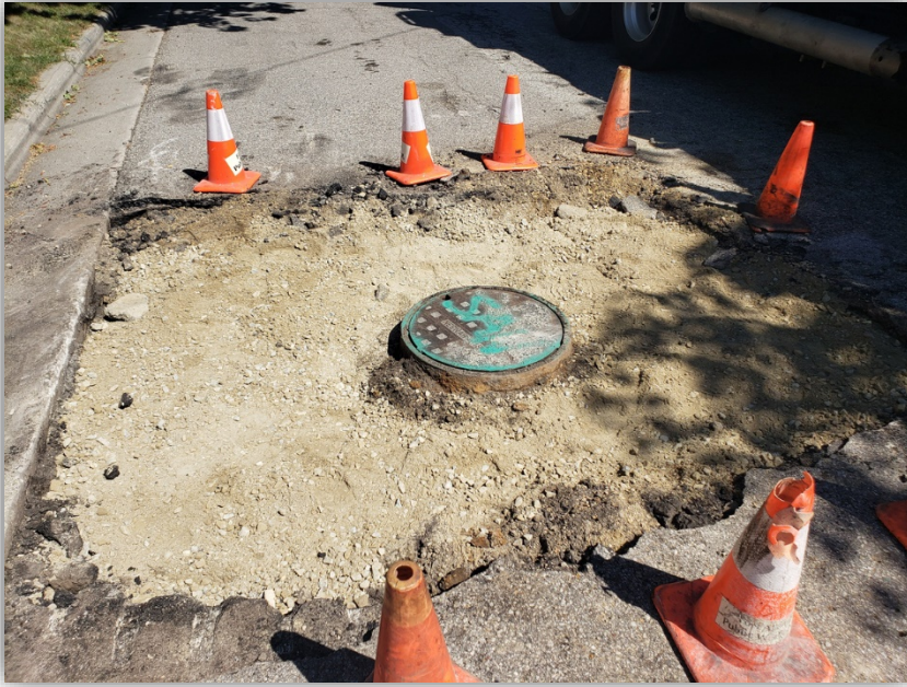
A REHABILITATED MANHOLE BEFORE CITY CREWS INSTALL ASPHALT PATCHING
