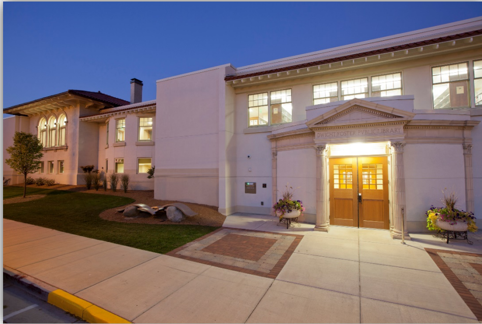
THE DWIGHT FOSTER PUBLIC LIBRARY, LOCATED AT 209 MERCHANTS AVENUE
