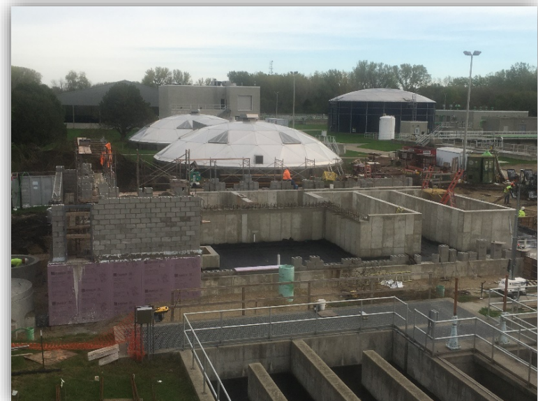
2021 CONSTRUCTION OF WASTEWATER TREATMENT FACILITY UPGRADES
