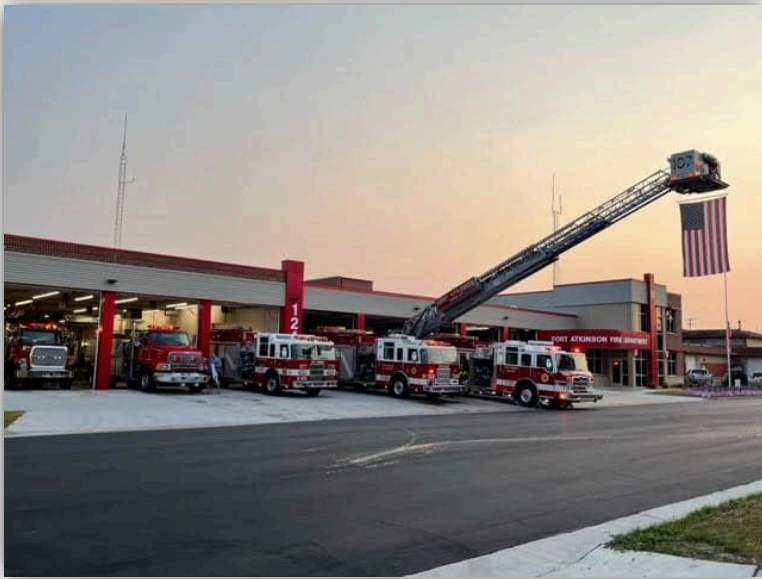
THE NEWLY RECONSTRUCTED FIRE DEPARTMENT MEMORIALIZES THE 20TH ANNIVERSARY OF THE SEPTEMBER 11TH TRAGEDY
