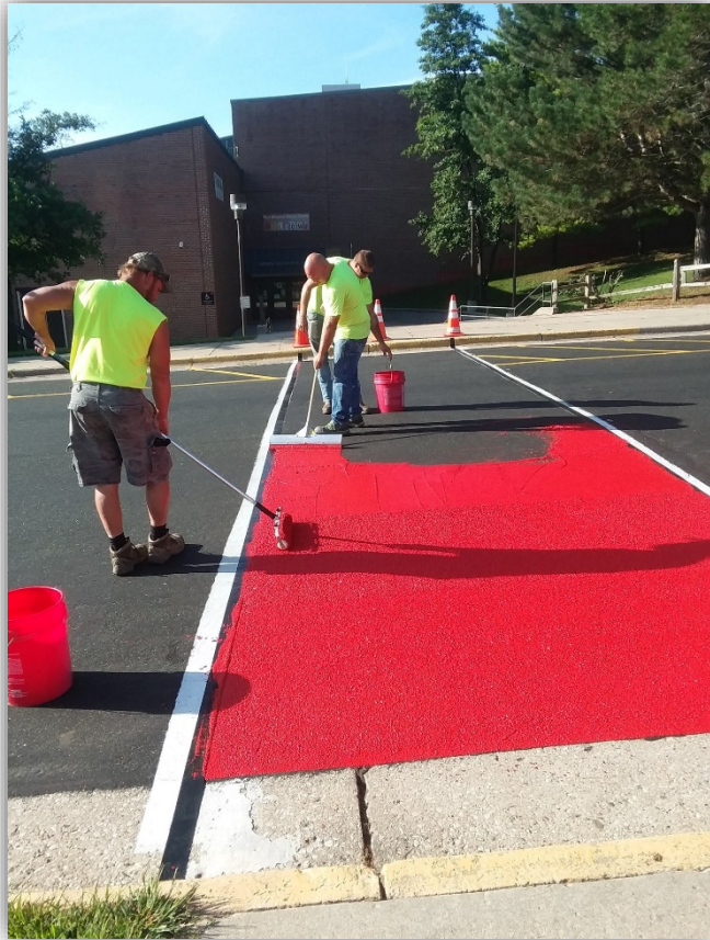
AN OPERATIONS CREW REPAINTS ONE OF THE CITY'S ICONIC RED CROSSWALKS
