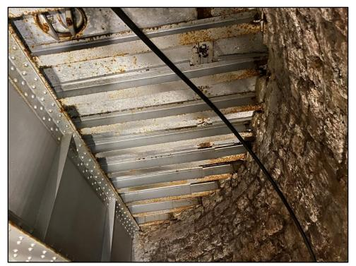
Photo 2: Steel beams below tank
