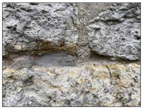
Photo 24: Different types of mortar
