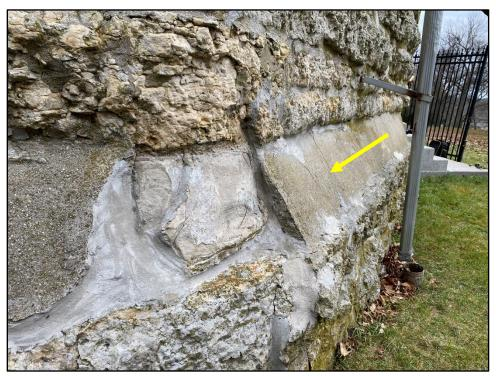
Photo 30: Cracked and missing concrete/mortar wash
