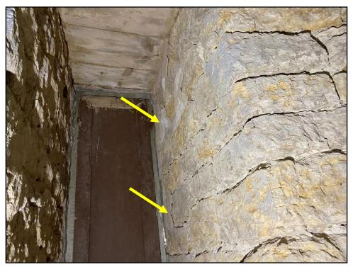
Photo 19: Spalled stone on "door" walls
