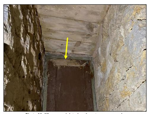
Photo 39: Minor wood deterioration at access panels
