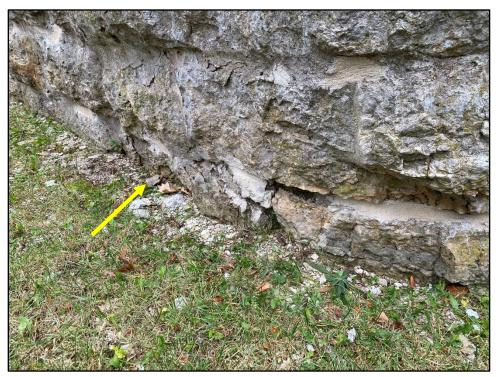
Photo 21: Stone deterioration at base of wall
