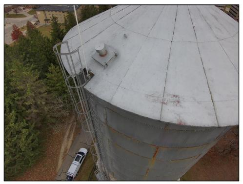
Photo 9: Exterior ladder to tank
