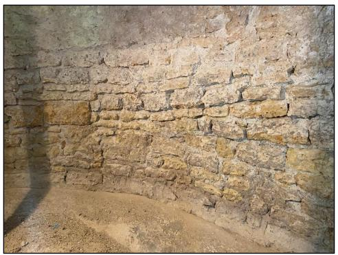
Photo 28: Deteriorated joints on interior – dust on floor is deteriorated mortar
