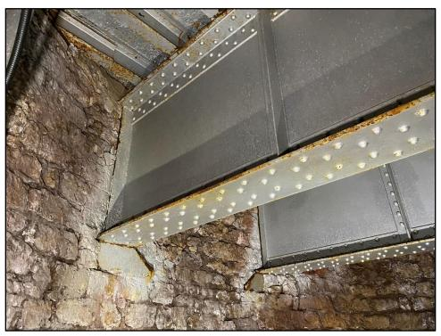
Photo 3: Steel plate girder supports
