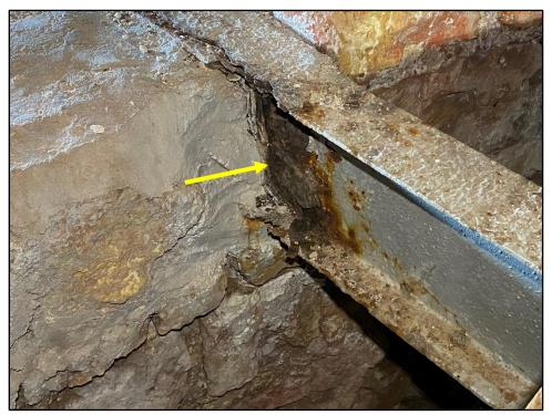
Photo 35: Corroding floor beam at exit to exterior platform
