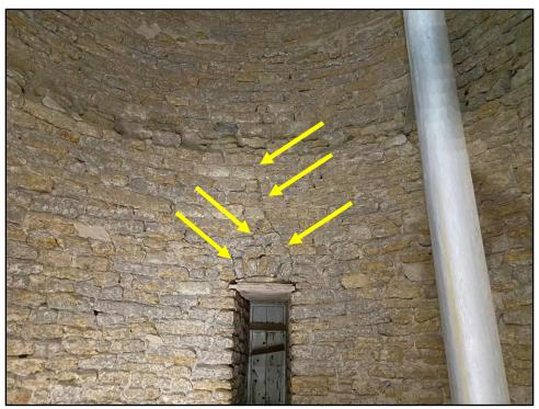
Photo 29: Crack on interior of tower
