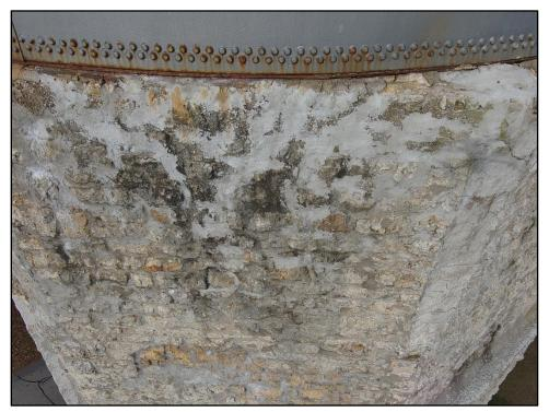
Photo 27: Repointing mortar at top of tower
