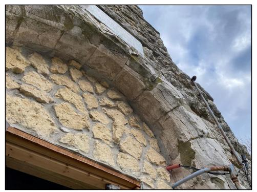
Photo 23: Cracked stone in entryway arch
