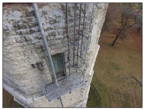
Photo 8: Exterior platform and ladder to tank
