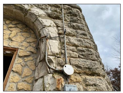
Photo 22: Cracked stone in entryway arch
