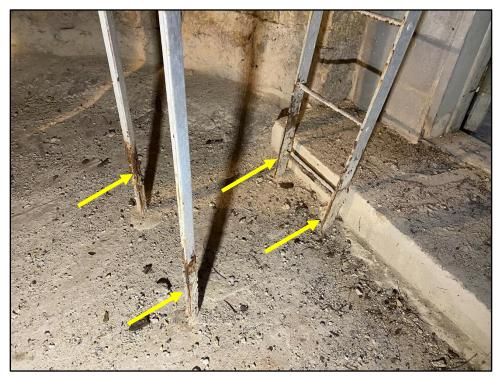
Photo 38: Base of interior ladder - corrosion on all pieces
