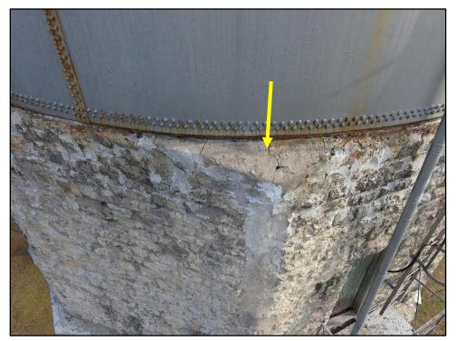
Photo 16: Deteriorating mortar wash at top of wall
