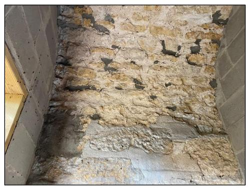
Photo 25: Different mortar at entry arch
