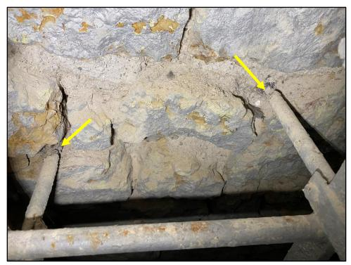
Photo 37: Corroded ladder connections at wall
