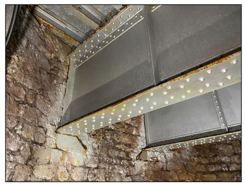
Photo 31: General light corrosion on support structure
