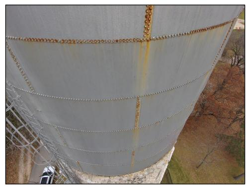
Photo 36: Rust staining on exterior of tank
