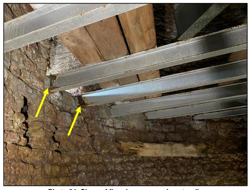
Photo 34: Signs of floor beam corrosion at walls
